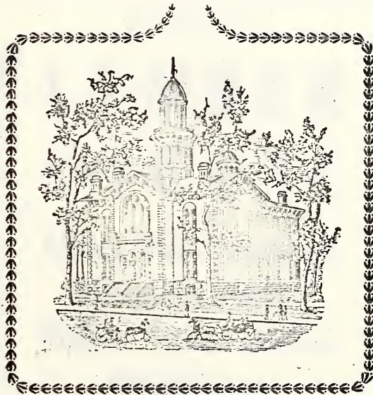
BUREAU COUNTY COURT HOUSE.
